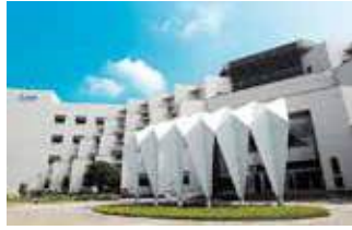
Tainan Plant (Diamond-rated Green Building)
